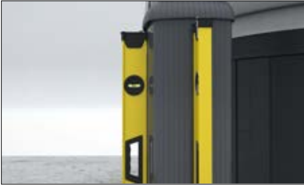
FIGURE 47: CHECK IF POSTS ARE STILL LEVEL
