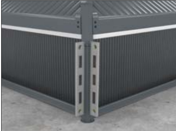
FIGURE 24: CHECK IF POSTS ARE LEVEL
