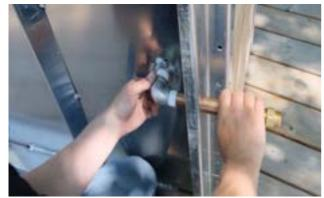
Thread the long piece of pipe into the elbow.
