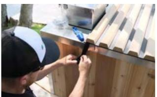
Place a locking clasp onto one of the straps at the end with the heater and pull it snug.
